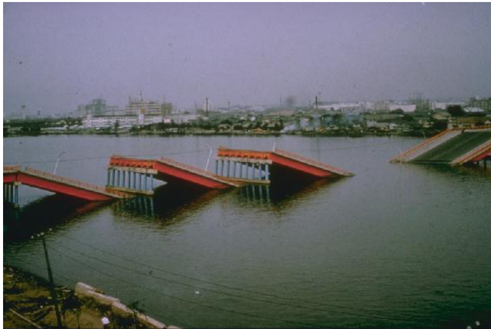
Figure 1-1 Lateral Spread Collapsed the Showa Bridge, Niigata, Japan. The City Suffered Slight Damage from Shaking, But Heavy Damage from Liquefaction (NRC, 1985).
